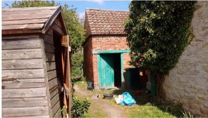
Fig 12 Outbuildings create enclosed character around access to cottage
