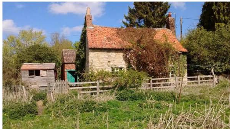
Fig 11 Church Lane Cottage from the south from the application site
