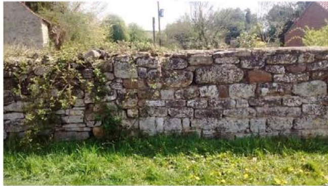
Fig 5 Dry stone wall bounding site to west with telegraph poles and trees beyond
